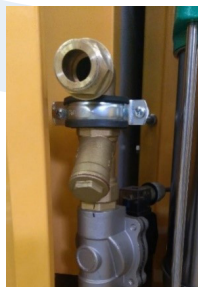
Loosening the filter nut
