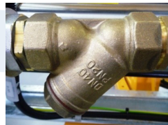
Loosening the filter nut
